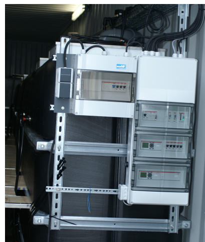
Electronic control unit of the waste water treatment system
