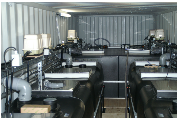
View into the interior of the container. A footbridge between the rows of tanks enables trouble-free work at the blowers fixed above the tanks. It also guarantees access to the membrane modules which are installed in the tanks.
