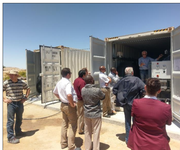
Training off he staff during first commissioning.
