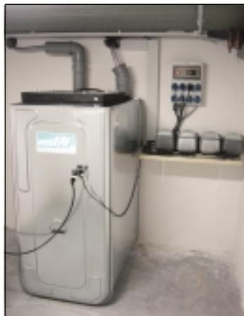
Installation of plant type MF-G-HKA 4 in a garage in combination with an existing septic tank
