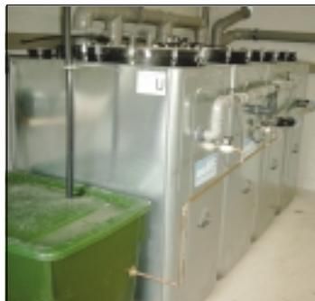
Plant type MF-HKA 8 for 8 inhabitants installed in the basement of the house
